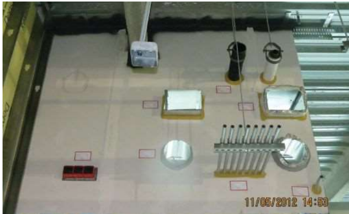
Firestopping mock-up. Corey Zussman photo
